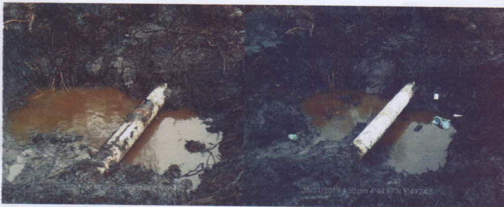
Pic 3. Repair work
