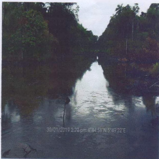
PIC 1. Before Excavation
