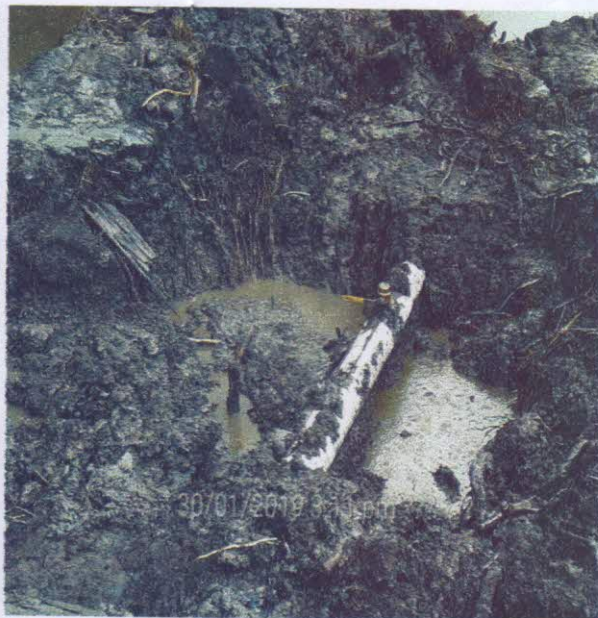
Pic 2. Installed 3" Valve
